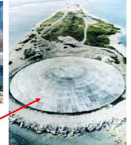
Runit dome, nuclear coffin, built in the 1970s. The US put nuclear waste under a dome. Now the dome is cracking and could be leaking nuclear waste.
